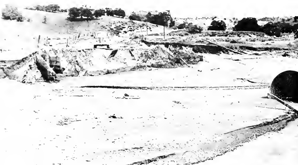
Realignment by-passes this washout of culvert and bridge
